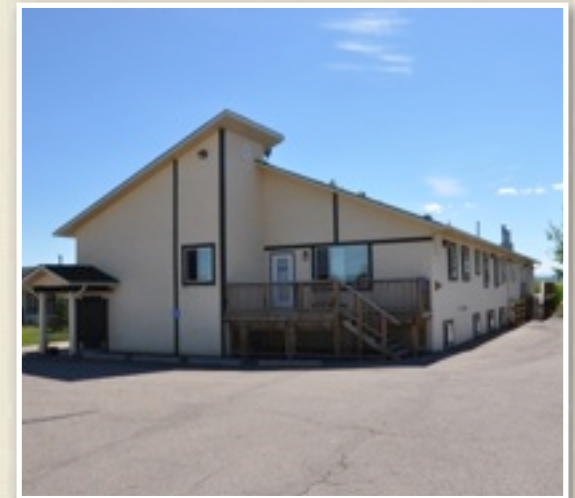
Built in 2003-2004, and dedicated in early July, 2005, the Mission Centre houses hundreds of people each year!
